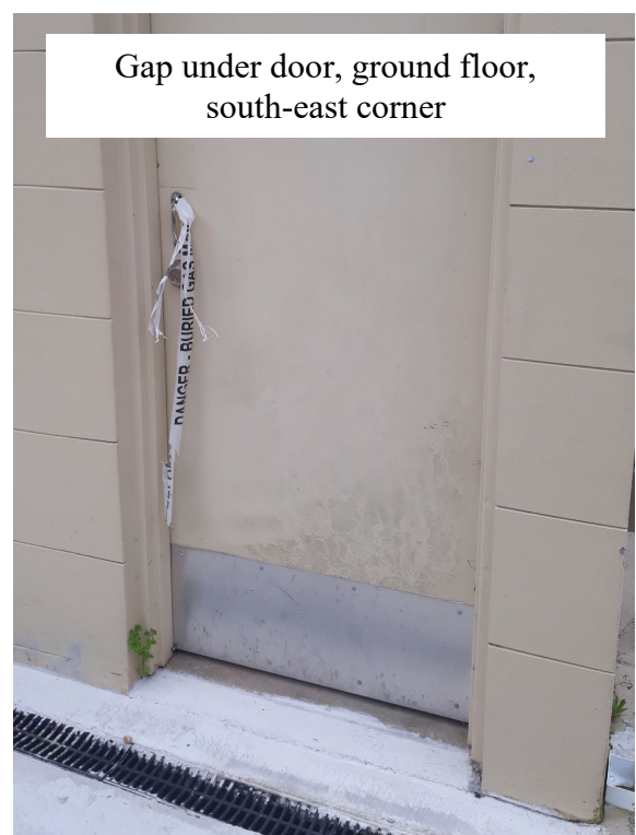
Figure 1: Examples of gaps around doors and windows.
